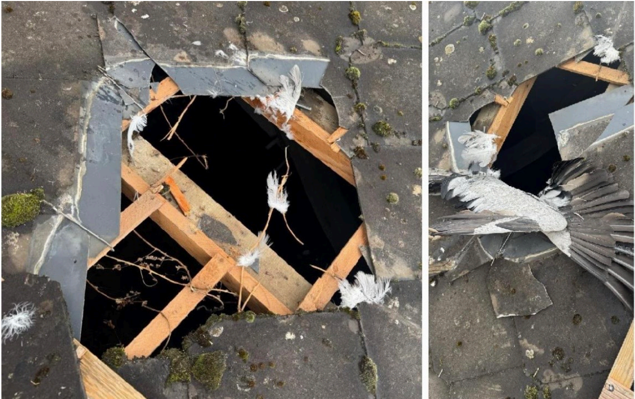
Image nº 85: A crane which crashed onto a roof in France. Info: LPO.
